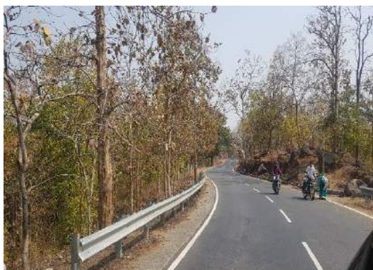
W Beam MCB at approaches at Km.13+500
