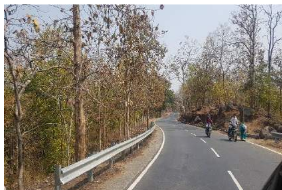
W Beam at approaches at Km.13+300
