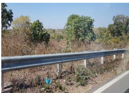
W Beam at approaches of MNB at Km 51+070
